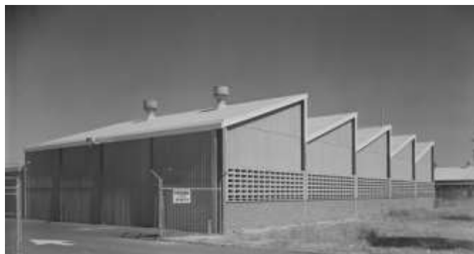
Wembley Technical School, Salvado Road, Wembley of 1962 (SLWA 340,566PD)
